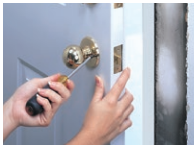
5 Install door hardware
