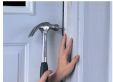
6 Install weatherstripped wood stops and replace interior trim
