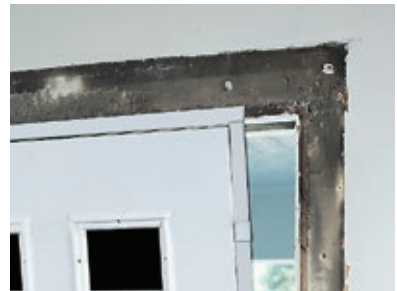
3 Insert the replacement unit into the opening from the interior side
