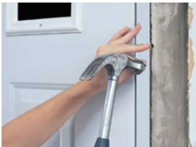
4 Nail replacement unit into position
